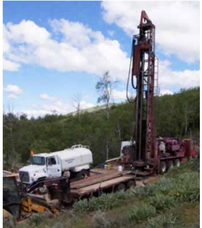
The BLM drills a groundwater monitoring well.
