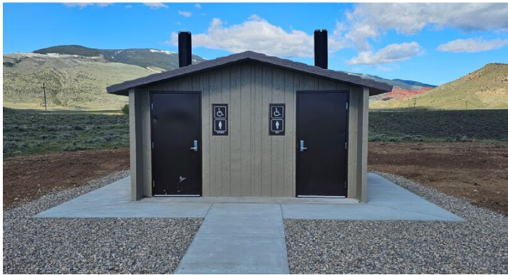
Concrete was poured at Outlaw Trails Vault Toilet
