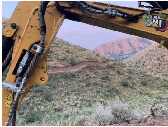
Hang Tight Trail Construction
