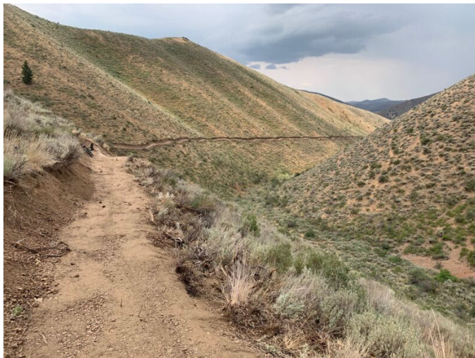
Future Trail Construction
