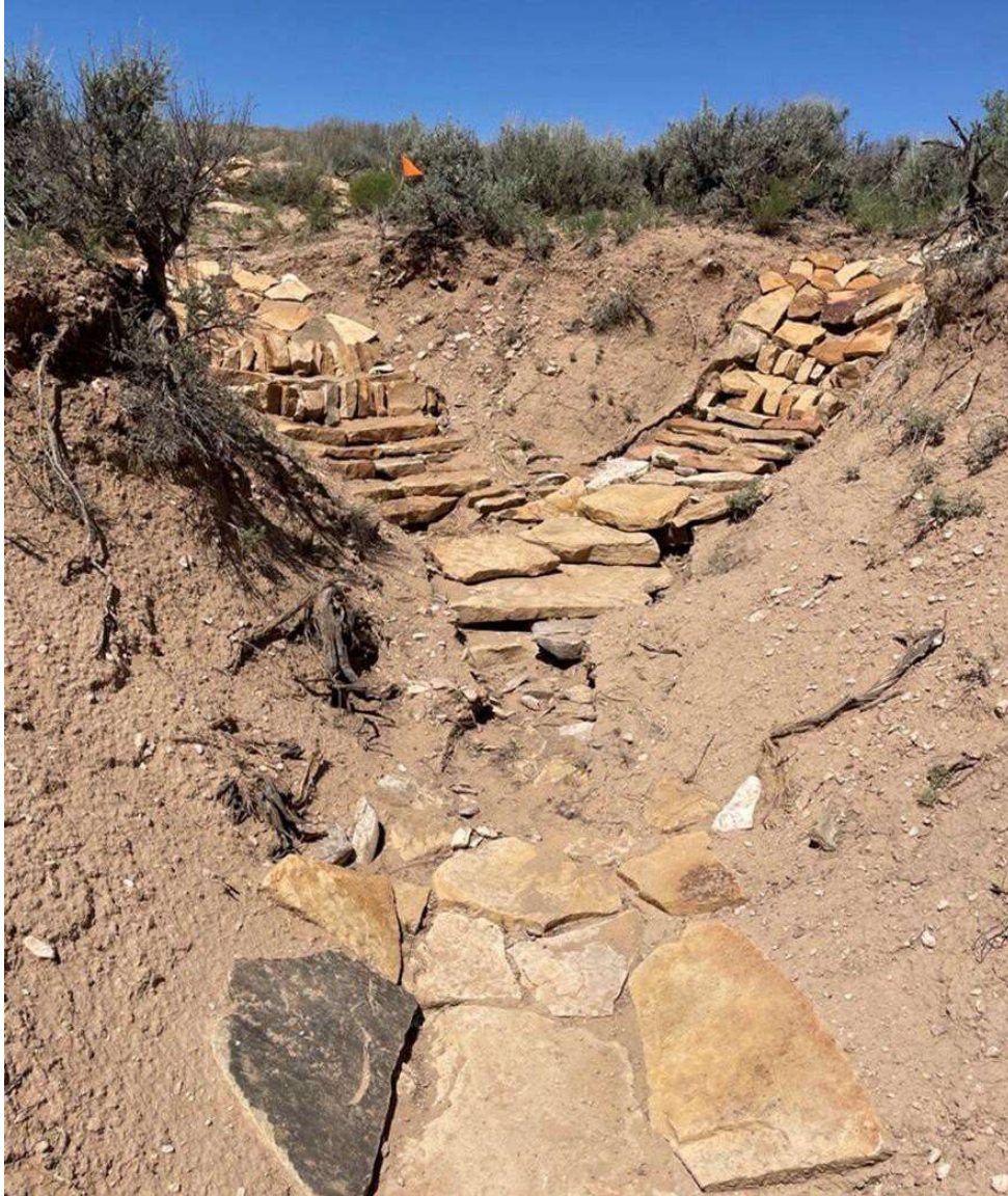
Zeedyke features constructed to improve wildlife habitat in Dry Creek Basin.
