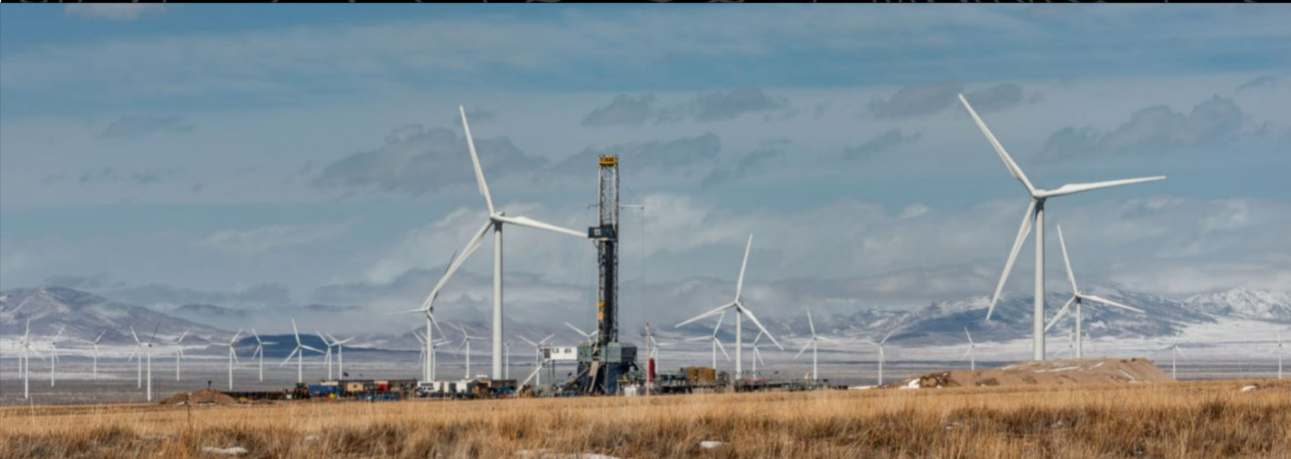
Fervo Energy Cape Geothermal power project (under construction), and Milford Wind project, Beaver County, Utah.
