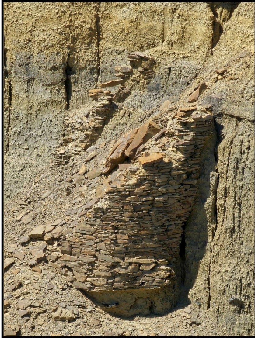
Figure 7: Masonry structure under threat from erosion
