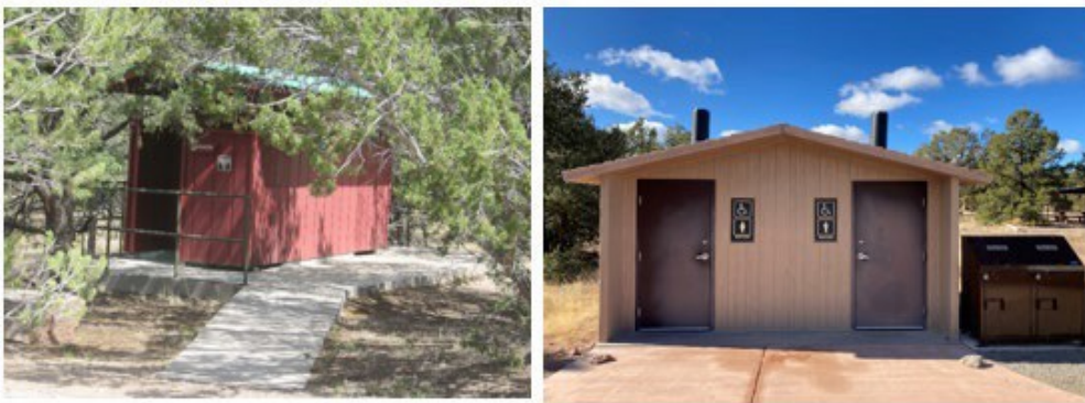
Figure 12: 2022 Vault Toilet Replacement
