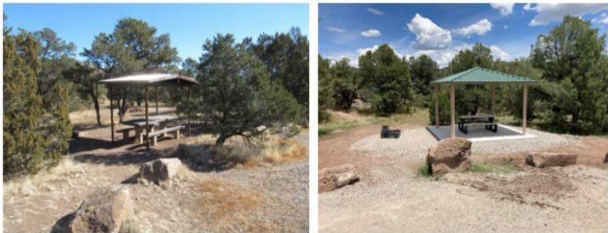
Figure 11: Before and after photos of facility upgrades in 2022
