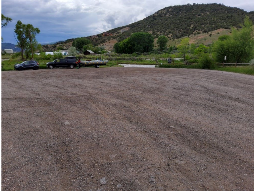
Dotsero Boat Ramp and Parking Area
