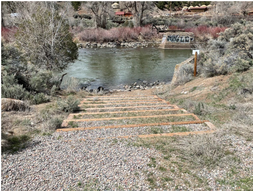
State Bridge Ramp #2
