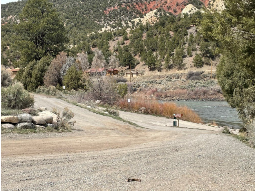
State Bridge Improved Ramp #1 Access and Area Turn-around
