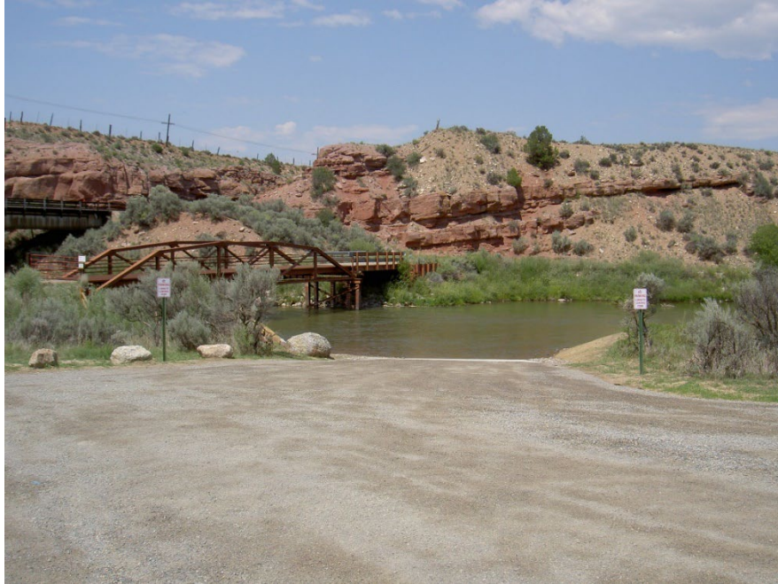
Two Bridges Site – Improved Boat Ramp
