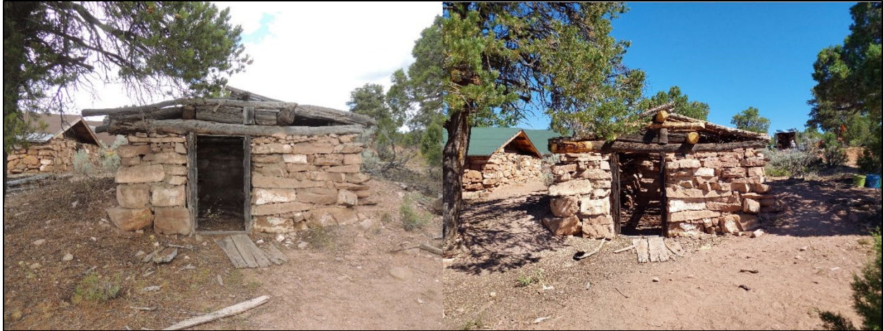
Figure 6. Before (2016) and after (2024) photos of Building 7.
