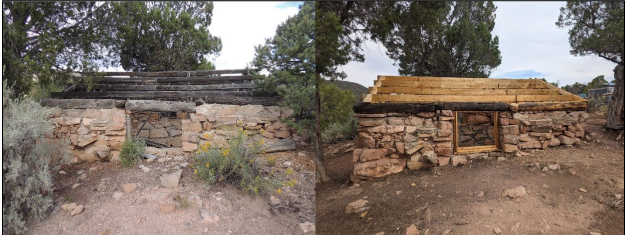
Figure 7. Before (2016) and after (2024) photos of the south side of Building 105..
