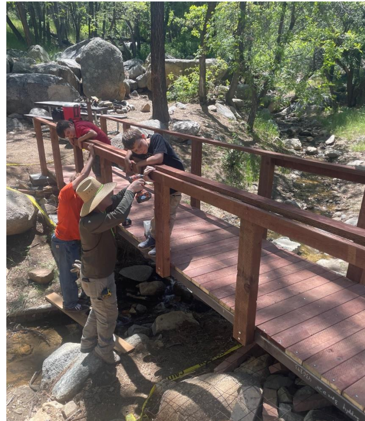
Scouts Construct New Pedestrian Bridge
