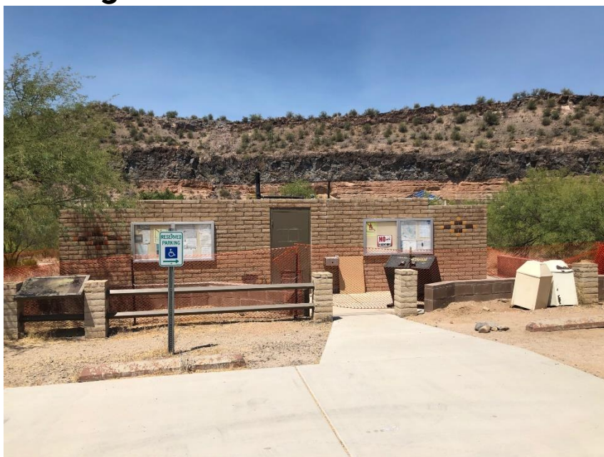
Burro Creek Campground Restroom During Renovation
