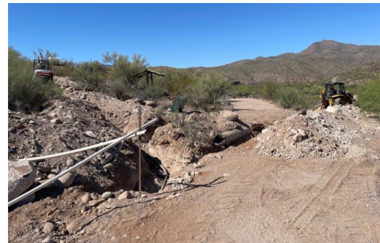
Waterline Renovation – Burro Creek Campground
