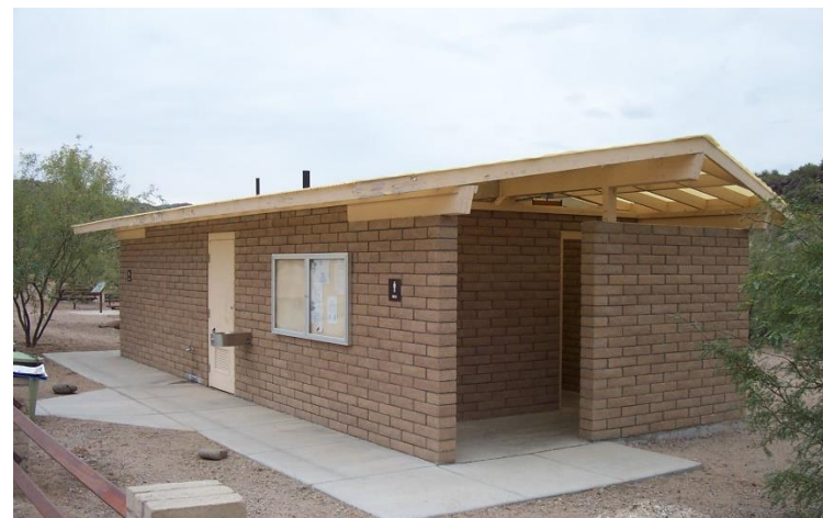
Lower restroom at Burro Creek before renovation
