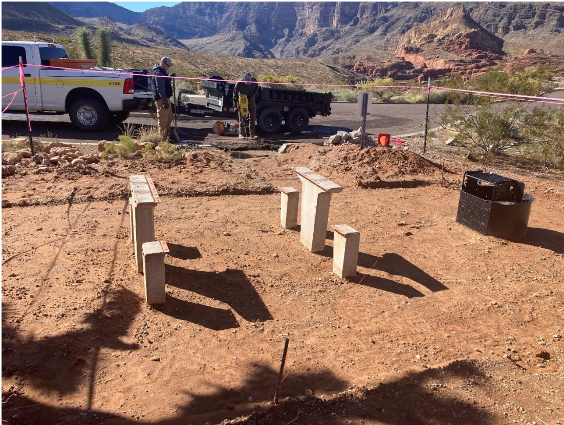
During Improvement Construction
