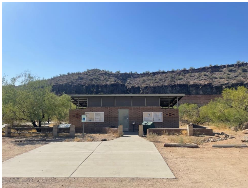
Burro Creek Campground Restroom After Renovation
