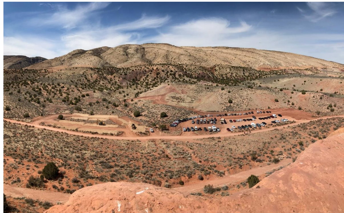
After Site Improvements
