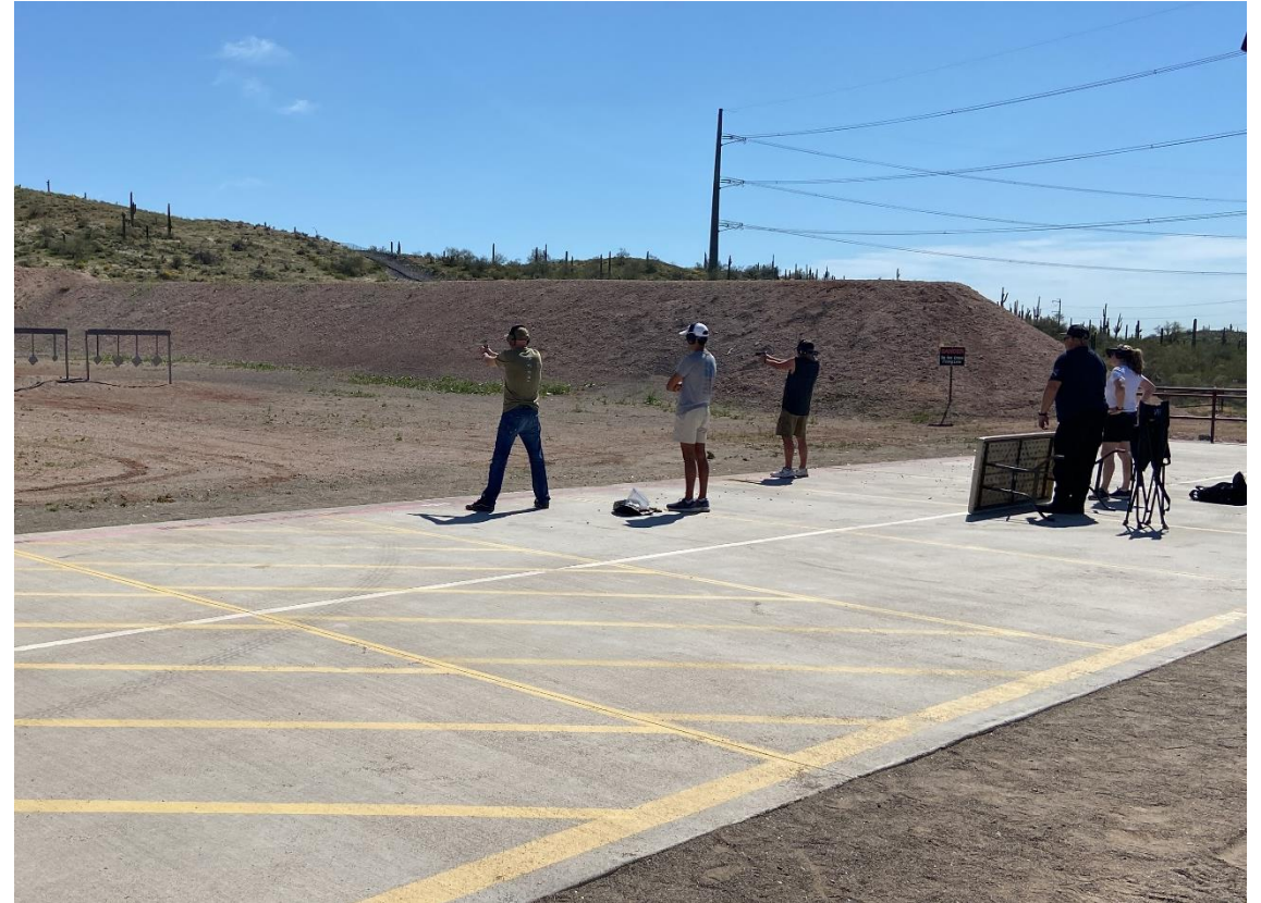
After Site Improvements
