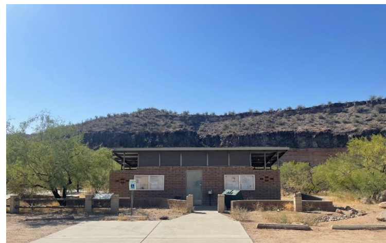
Lower restroom at Burro Creek after renovation
