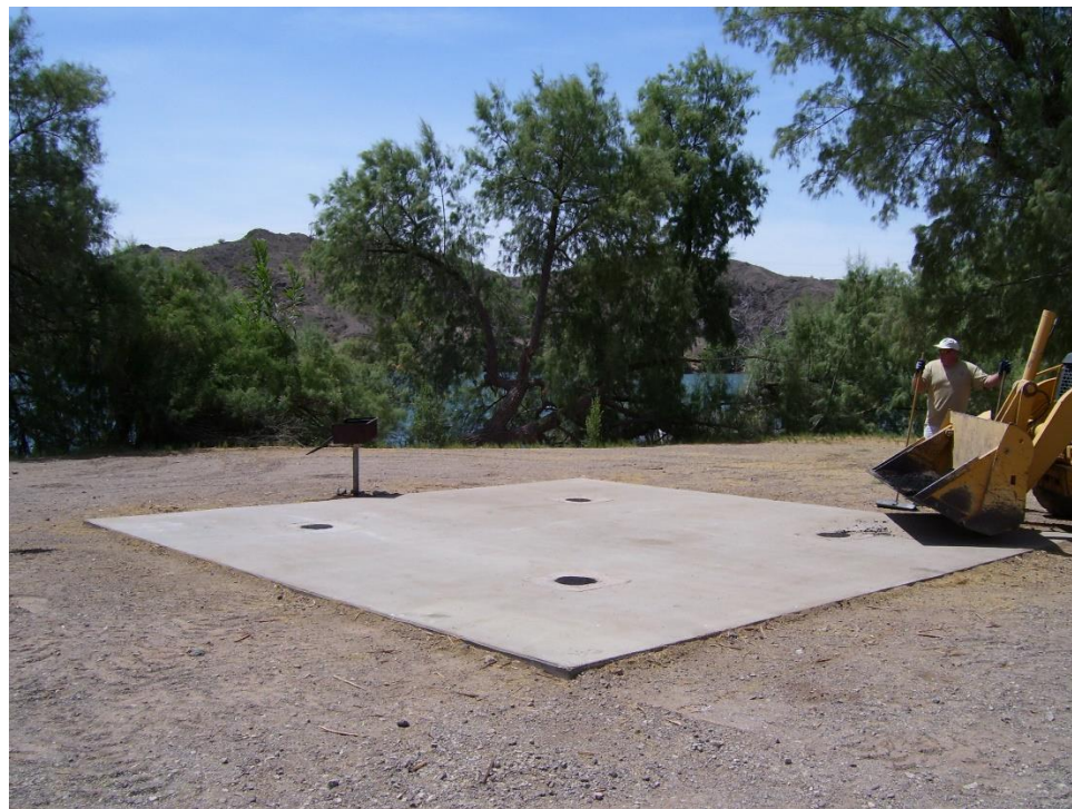
Staff replace a ramada at Crossroads Campground
