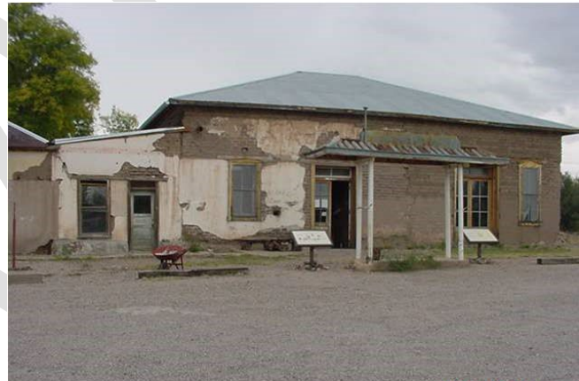
Figure 17: Historic mercantile building at the Fairbank Townsite
