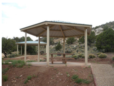
Figure 3: Shade Structure at Campsite Area
