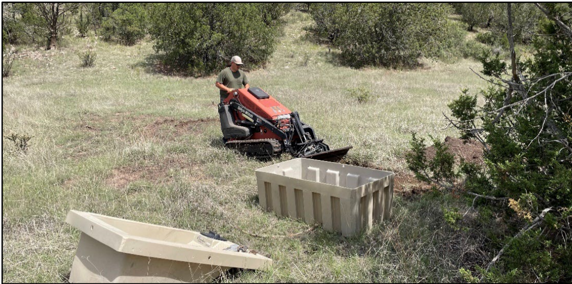
Using a trail dozer, BLM installs a wildlife waterer at the Conservation Area.
