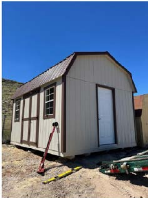
New structure being placed
