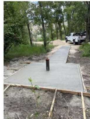
Construction of well pad access
