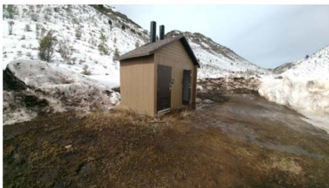
Restroom at Pine Creek Winter Trailhead
