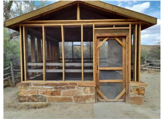
Sand Wash Screen Shelter Improvements
