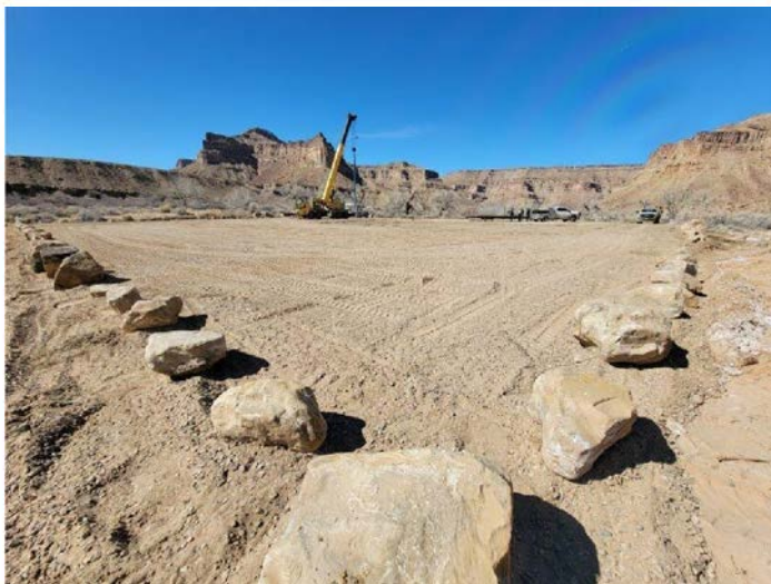
Boat Ramp Parking Expansion (Phase 3)
