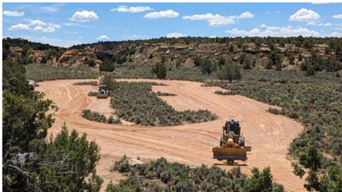
Development of the Tilted Mesa MTB trailhead.
