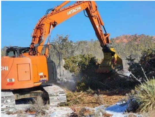
Machinery clearing vegetation for expansion
