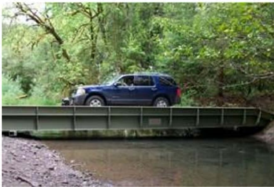
Temporary bridge at Edson group site.
