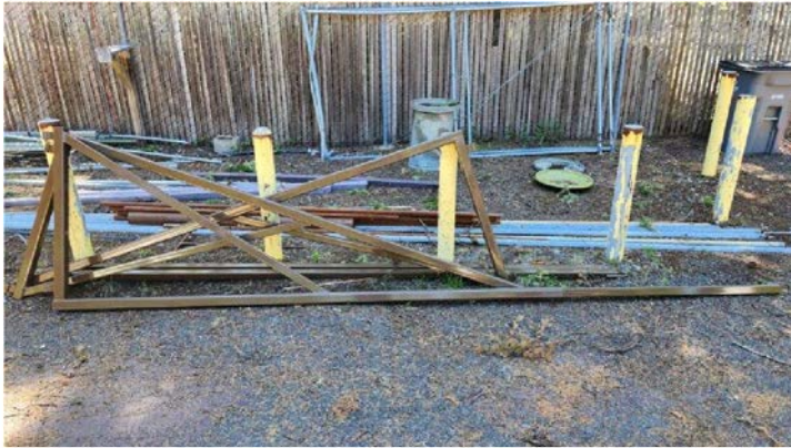
New gates ready for installation
