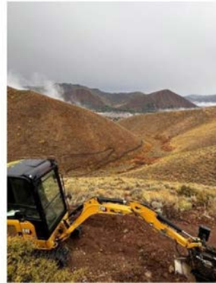
Silver lining trail construction
