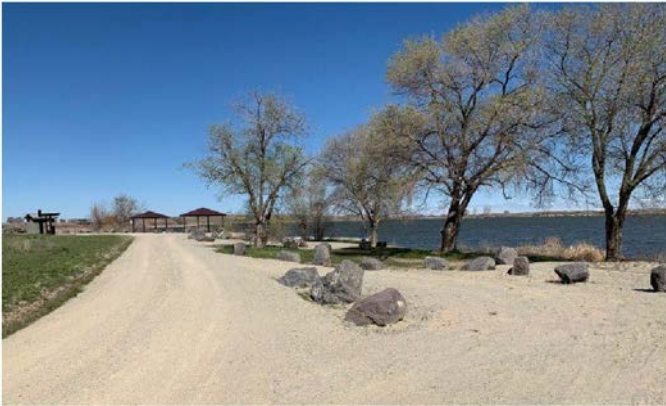
Wilson Lake Campground Construction
