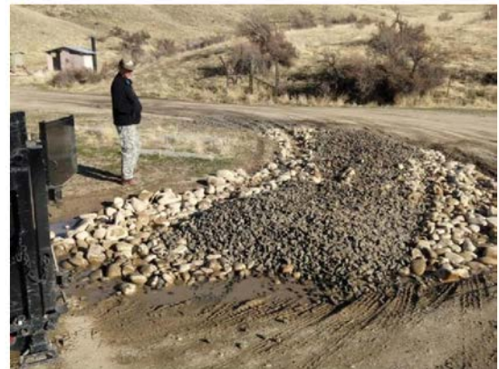
Engineering/Ops/Recreation Repair Pothole
