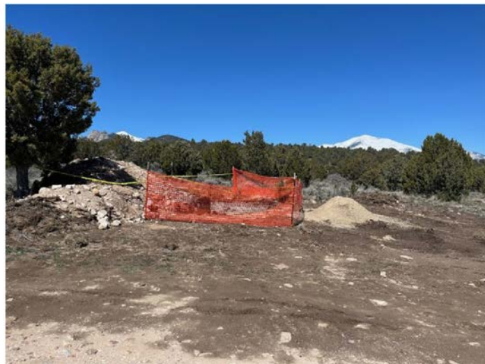
Construction of new CXT Toilet at Pinyon Pine
