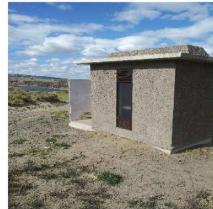
Refurbished CXT toilet at Salmon Creek Reservoir
