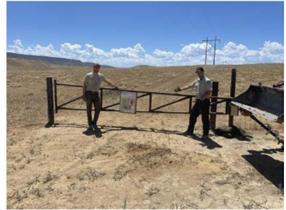
BLM rangers installing gate to protect buckwheat
