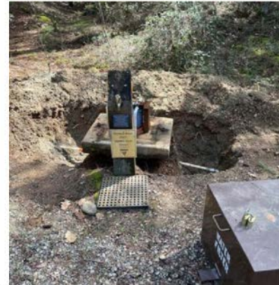
Water Spigot Valve Replacement and Pipe Repair
