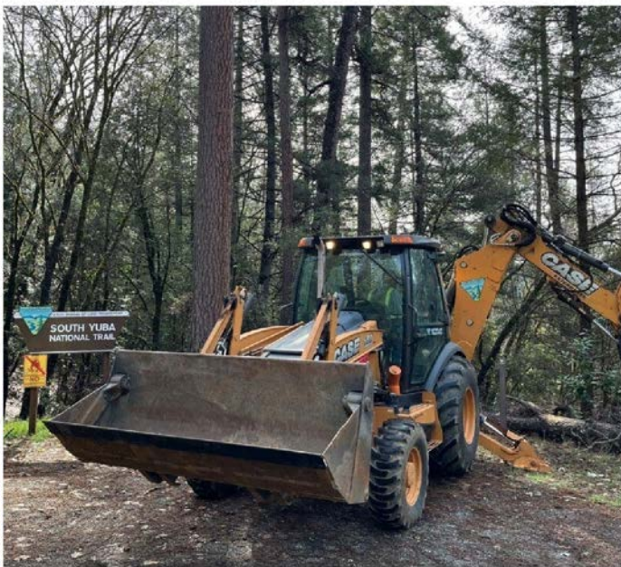
Fuels and Hazard Tree Work at S. Yuba Campground
