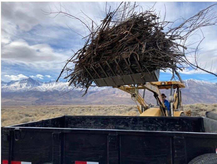
Improving campgrounds with heavy equipment.
