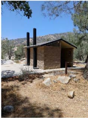
Vault toilet at the Keysville Boat Launch
