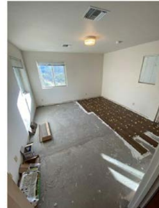
Installation of new tile in living quarters
