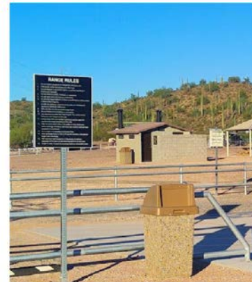
Church Camp Recreational Shooting Sport Facility
