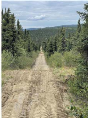
Repaired Rolling Grade Dips
