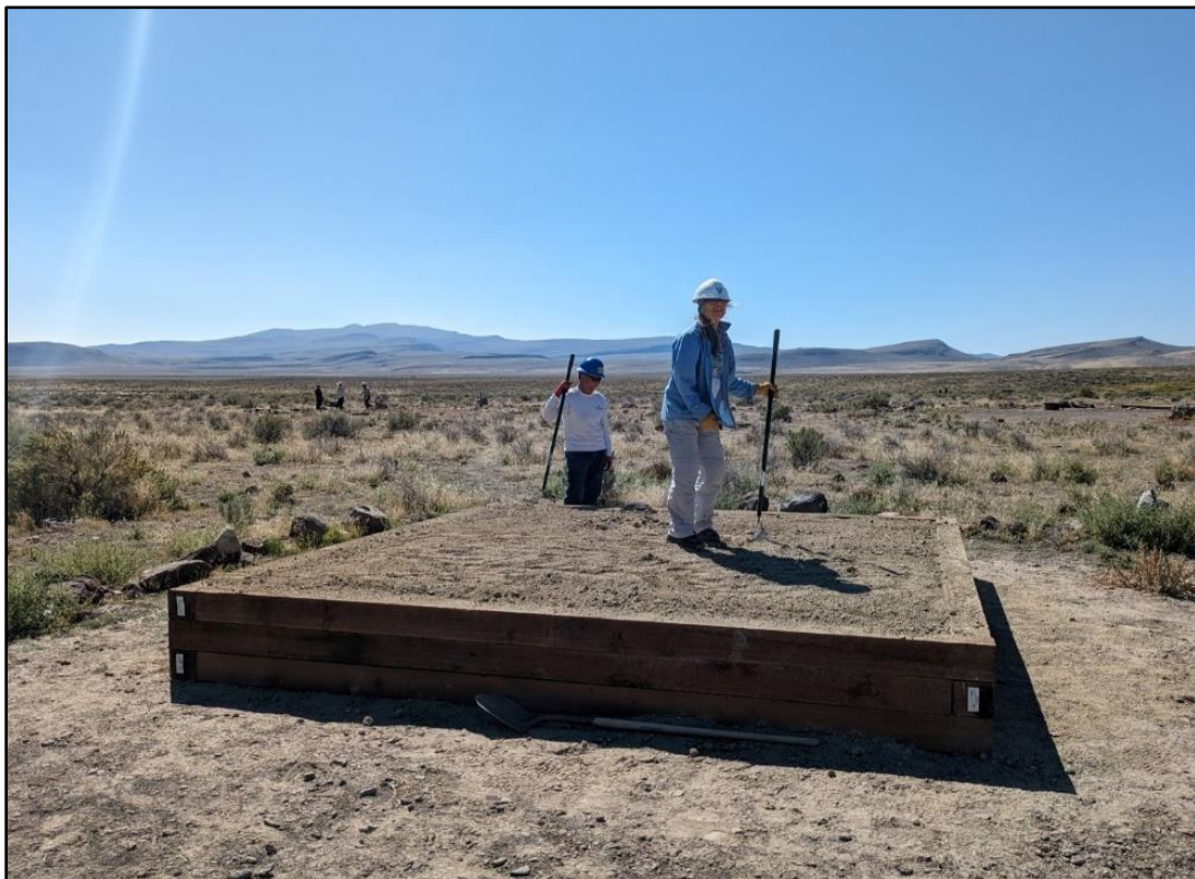
Figure 10. Volunteers help construct ADA tent pad in Soldier Meadows. Photo Credit: Megan Berner
