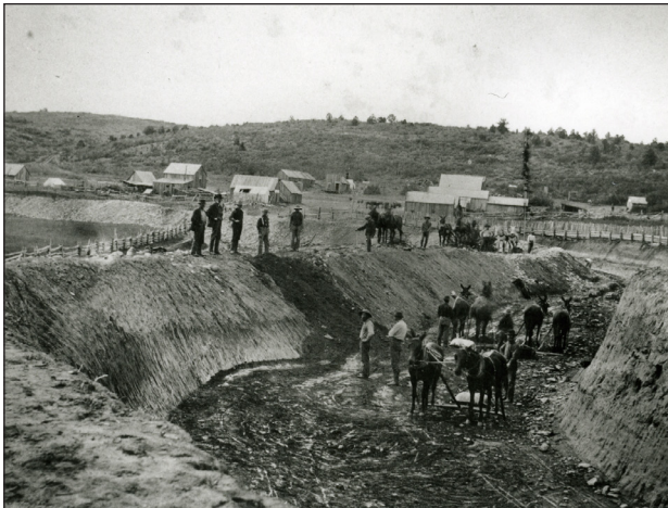
Digging a canal through Big Bend, 1887. Photo courtesy of Andy Harris
