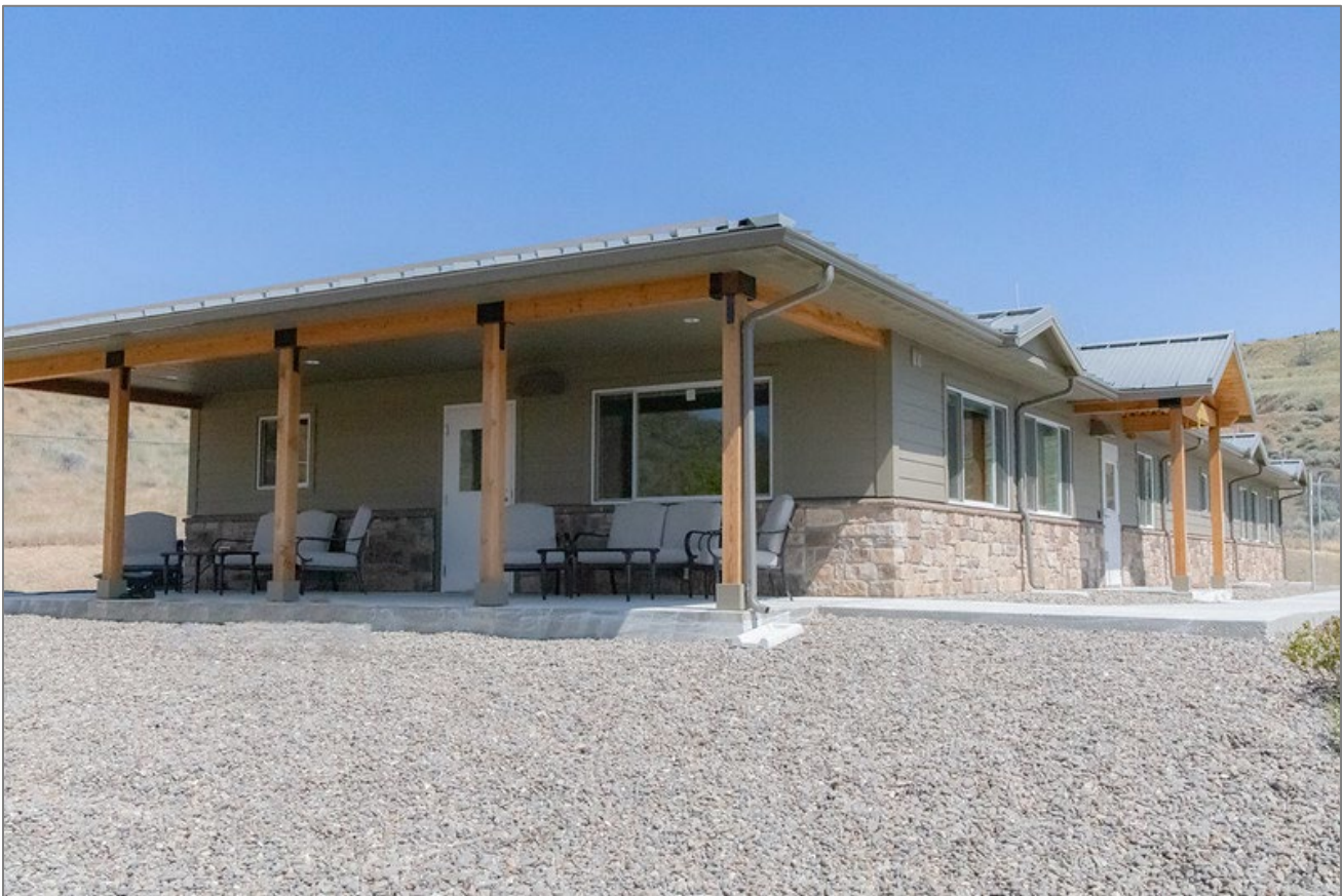
Seasonal housing in the Bakeoven facilities complex, Maupin, Oregon. Photo taken by Morgan Rubanow, BLM, on June 1, 2023.
