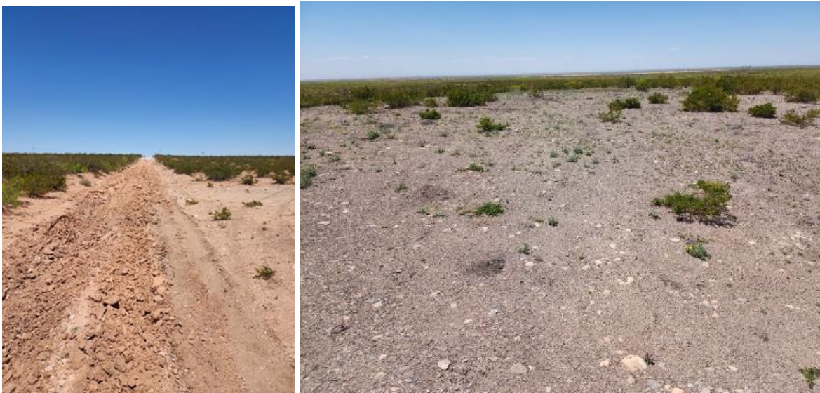
Photo 1 (left) showing county road after ripping for restoration; Photo 2 (right) show post-restoration results after seeding and revegetation.
