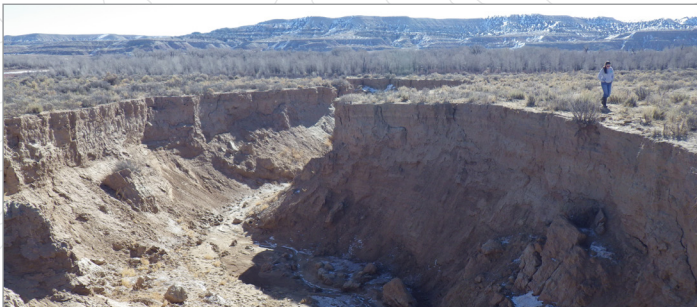
Blown-out and incised creek in need of restoration.
