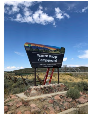
New portal sign installation at campground
