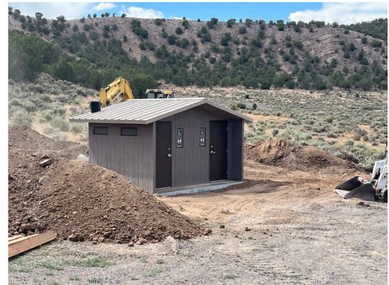
Vault Toilet at Saul's Meadow Campground
