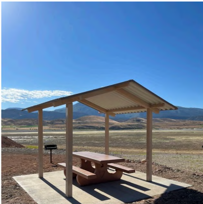
One of Two Shade Structures at Gunnison Reservoir
