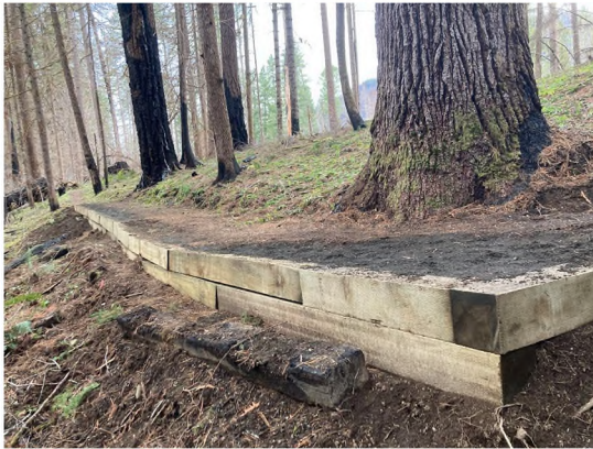
Retaining Wall Reconstruction
