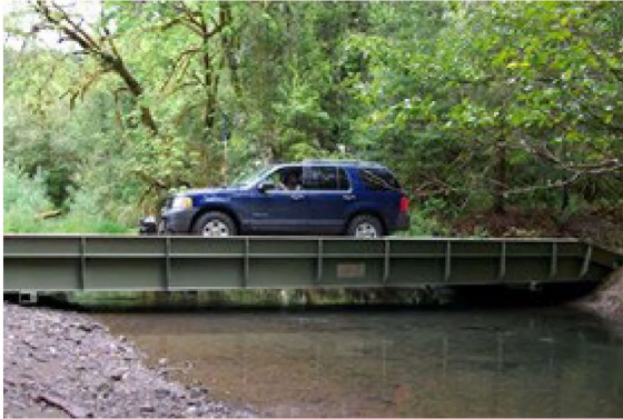
Edson Creek Campground bridge.
