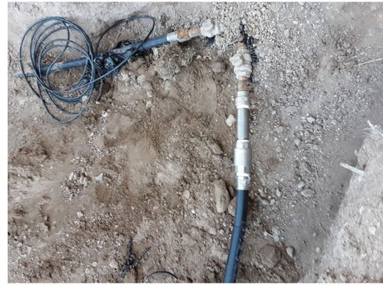
Potable water system upgrade
