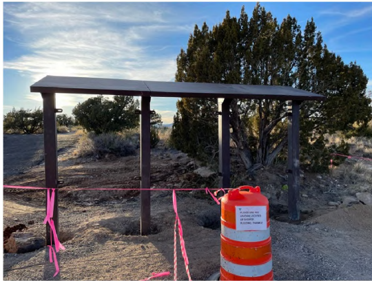
Installing Information Kiosk at Valley of Fires
