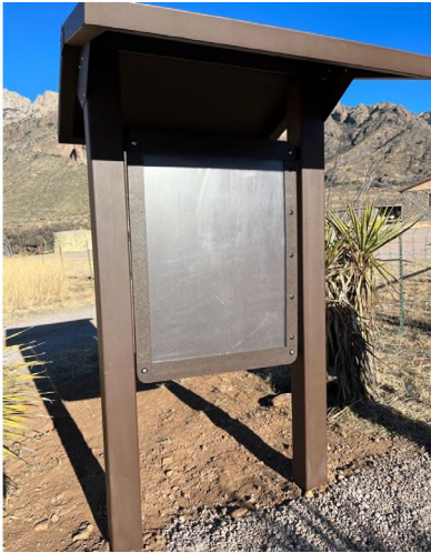
KIOSK AND INFORMATION PANEL INSTALLATION
