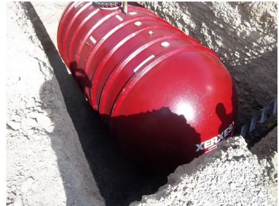
Water Tank at Rhyolite
