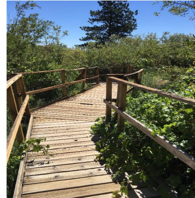
Current condition of Lost Creek Boardwalk
