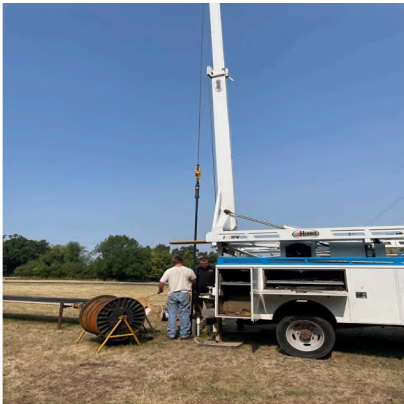
Well Rig Installing New Well Pump
