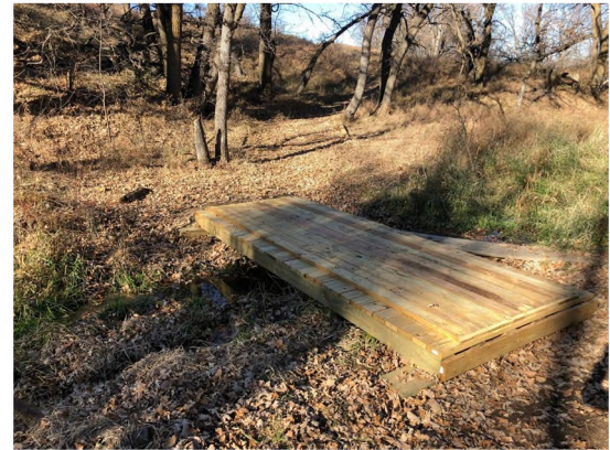
Trail Bridge at Schnell Recreation Area
