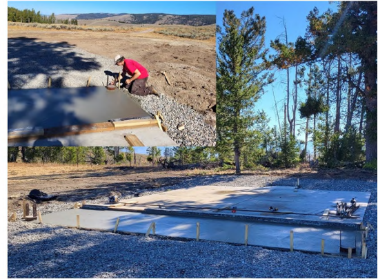
BLM employee finishing concrete foundation.
