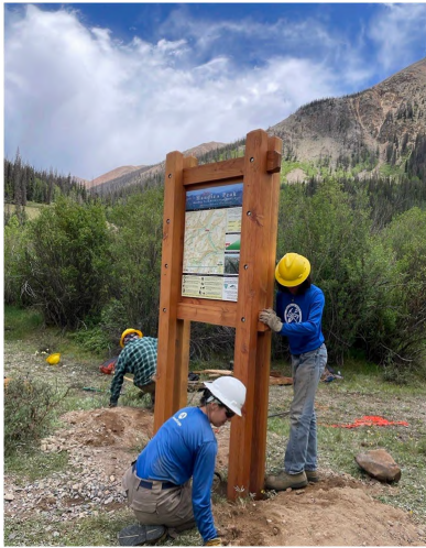
Wilderness Kiosk Installation
