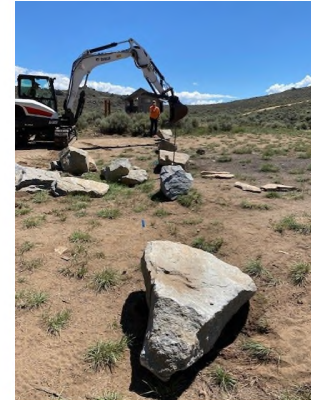
Excavator Placing Boulders to Delineate Parking
