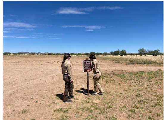
Youth crew installing a new group site sign
