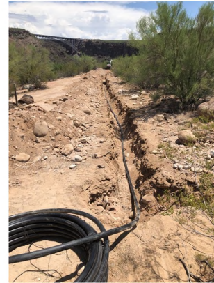
Contractor installs HDPE water line
