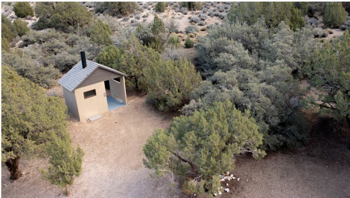
Vault Toilet at Lime Kiln Canyon Climbing Area
